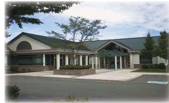
Highline Water District office
