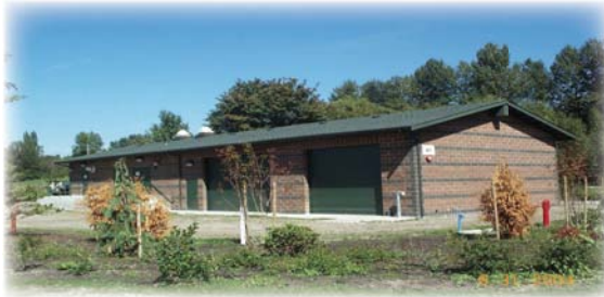
Tyee Treatment Plant
